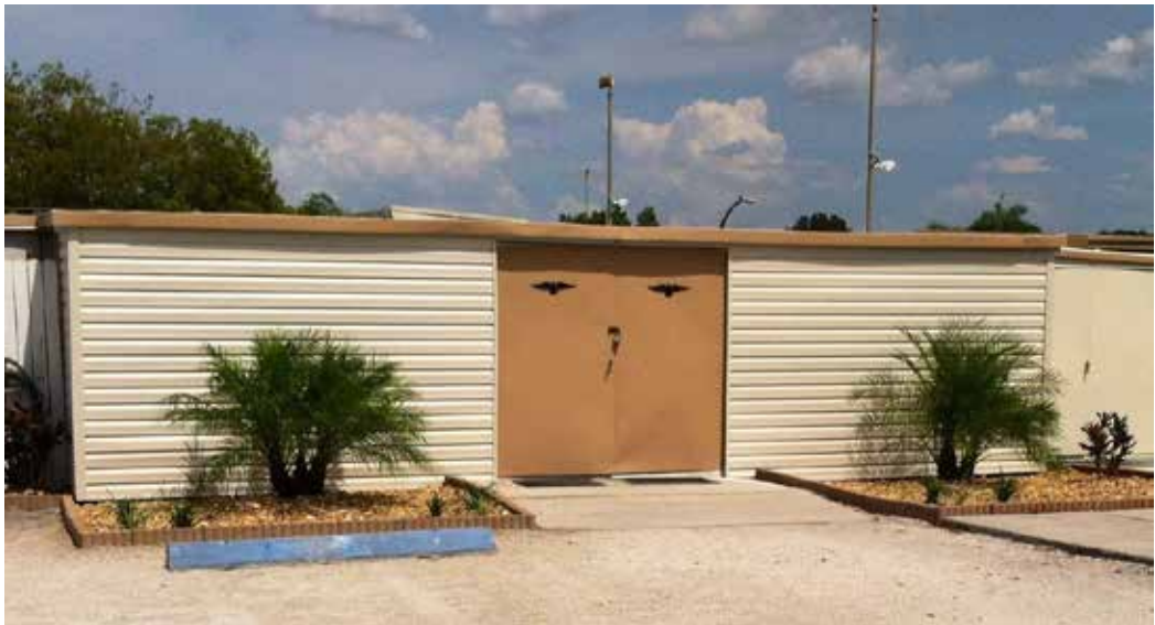
Shed remodeled - thanks, Clay!
